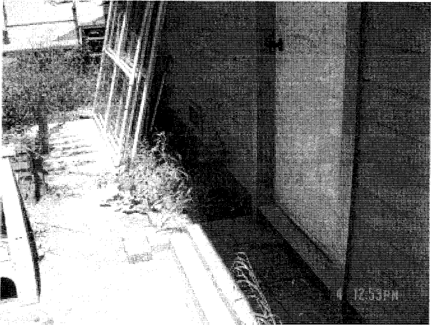
Back of Garage Addition, June 26, 2007
