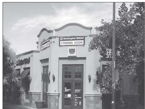
The newly constructed building on the corner of Mt. Diablo and Salvio Street will house a bank and space for retail use.
