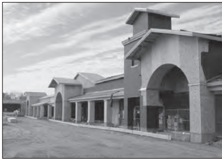
Renovation in progress at Olivera Crossing
