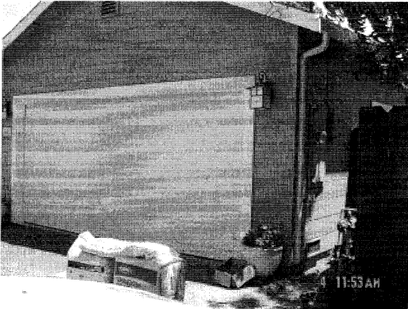
Front of Garage Addition, June 26, 2007
